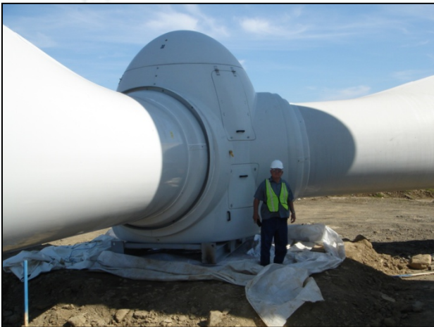
Assembled Rotor
