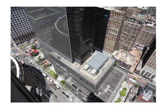
One Penn Plaza, 6MW natural gas CHP rooftop unit, provides more than half the required energy
